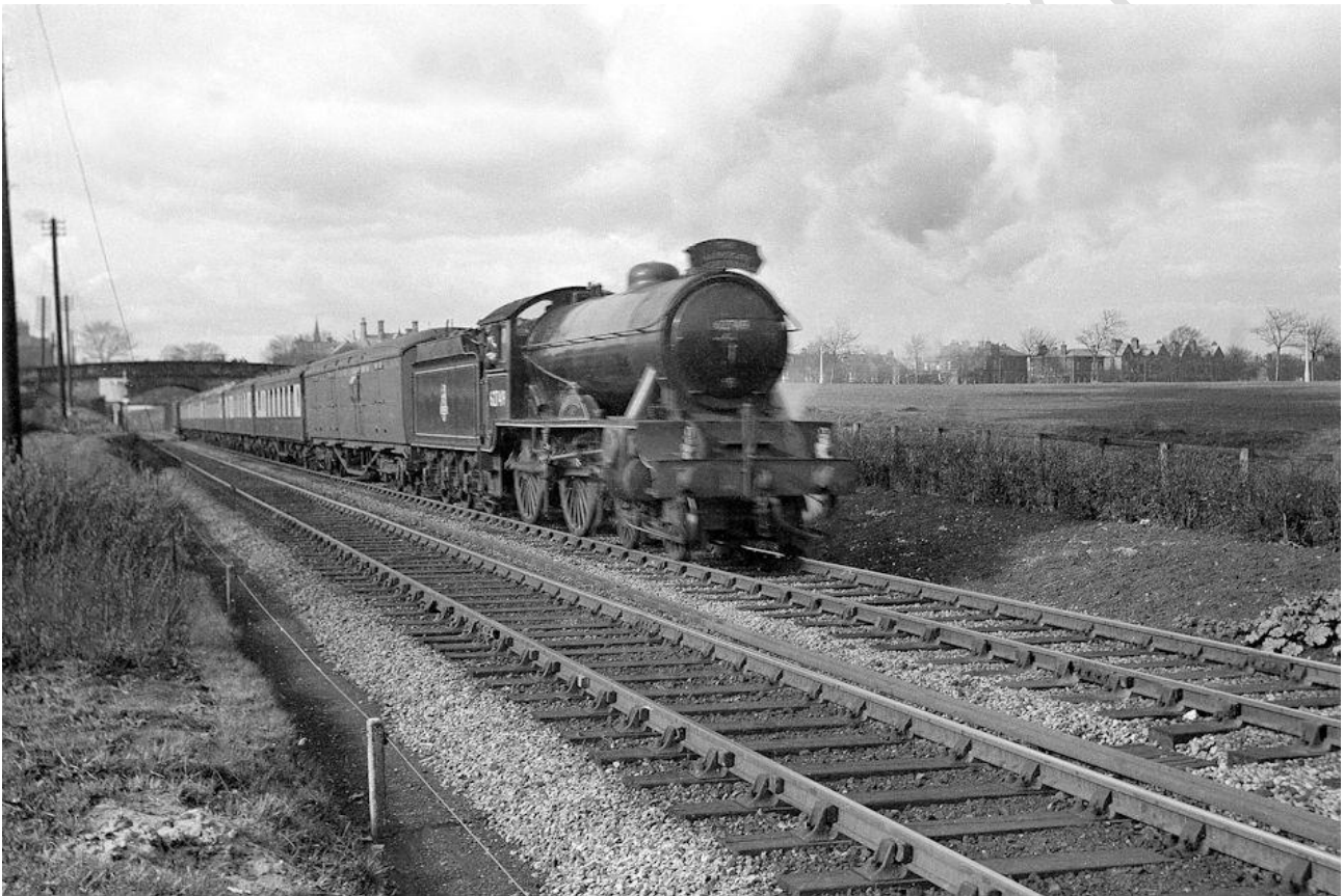
©Gerry Pierson Collection - The Armstrong Railway Photographic Trust.
