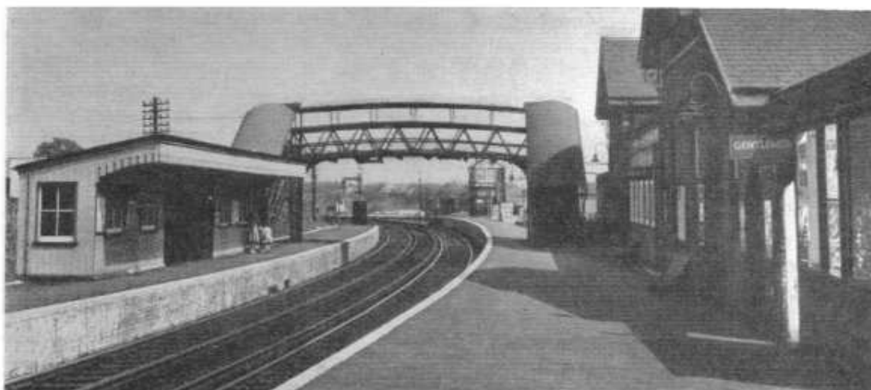
Bat & Ball Station, Sevenoaks, from the south
