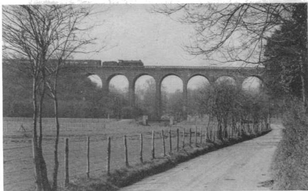
Dover to London train crossing Eynsford Viaduct in March, 1948, when Polhill Tunnel was closed for engineering works
